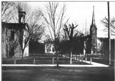
ST. MICHAEL'S CATHOLIC CHURCH, SCHOOL AND PRIEST'S RESIDENCE,
